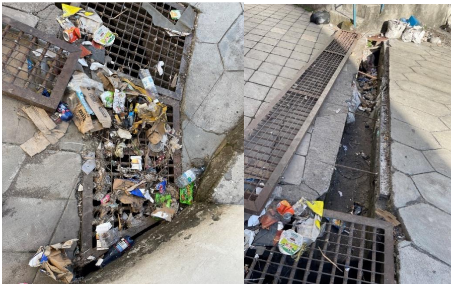
Figure 8: Rainwater drainage channel in Medina blocked by solid waste from the market.
